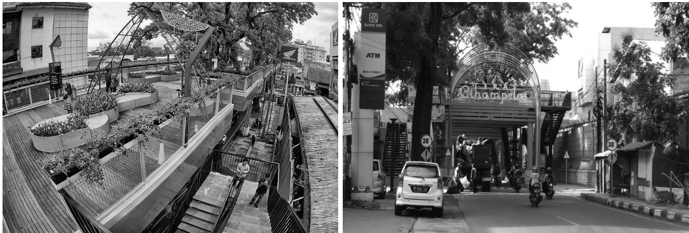
Figure 4.3 the Skywalk from above (left) and from the street (right) (Hotmaduma, 2017)
