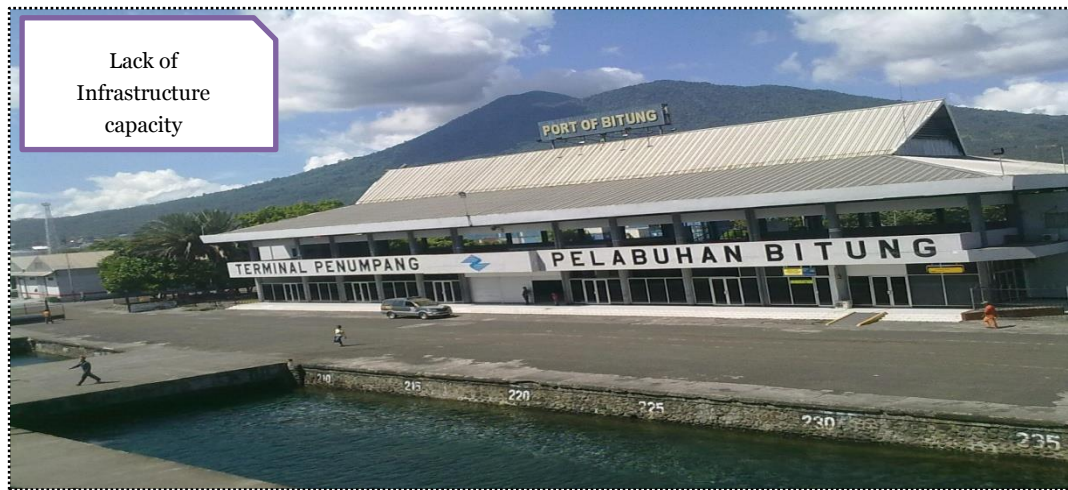
Figure 15 Passenger Terminal of Port of Bitung Source: www.bacatransportasi.com
