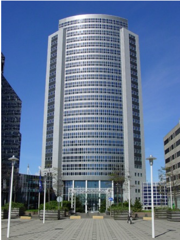
Crystal Tower. Location: Amsterdam, Sloterdijk
