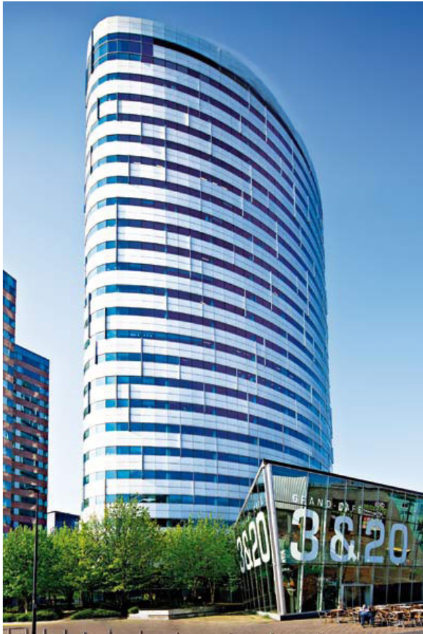
Oval Tower. Location: Amsterdam, South-East
