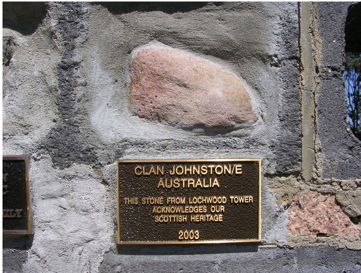
Figure 4.8 Stone dedicated by clan in 'Wall of History'
