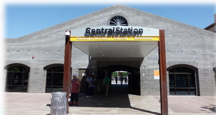
CENTRAL STATION IN DOWNTOWN PHOENIX
