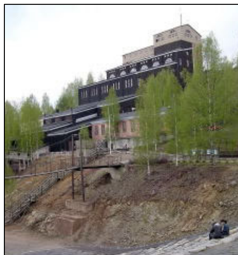
Figure 5.4 Outokumpu mine (picture by author)
