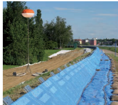
Figure 17: Inflatable dike in Dresden (Fischer, 2013)
