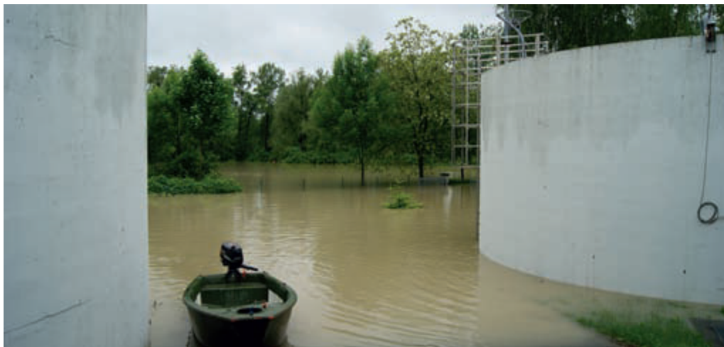
Figure 19: Settling tanks are high enough to endure a flood in Tittmoning (Fischer, 2013)
