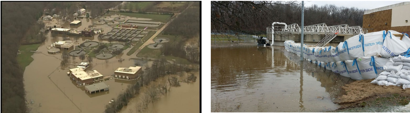
Figures 23 and 24: Grand Glaize Treatment Plant during the flood (SLMSD, 2016)
