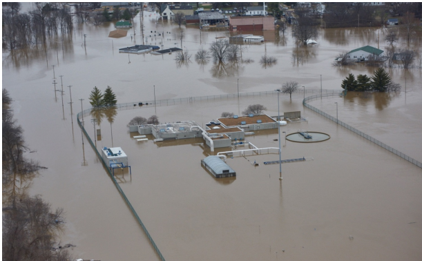
Figure 25: Fenton Treatment Plant during the flood (SLMSD, 2016)
