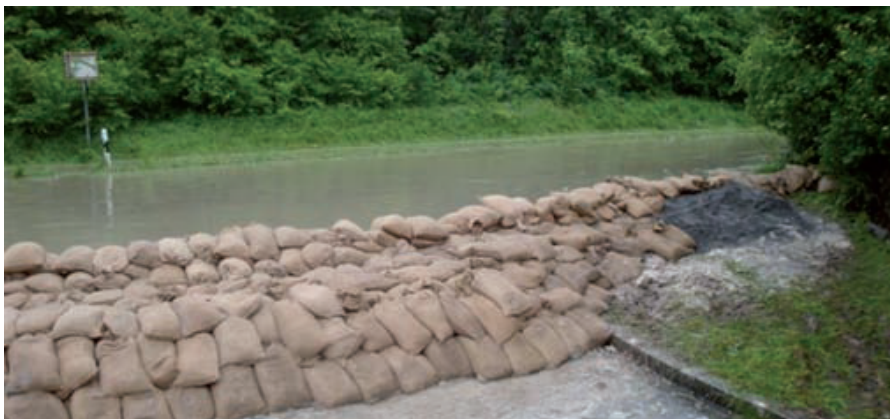
Figure 18: Emergency dike (Fischer, 2013)
