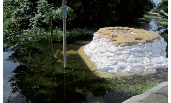
Figure 15: A pumping station protected by sand bags in Dömitz (Fischer, 2013)
