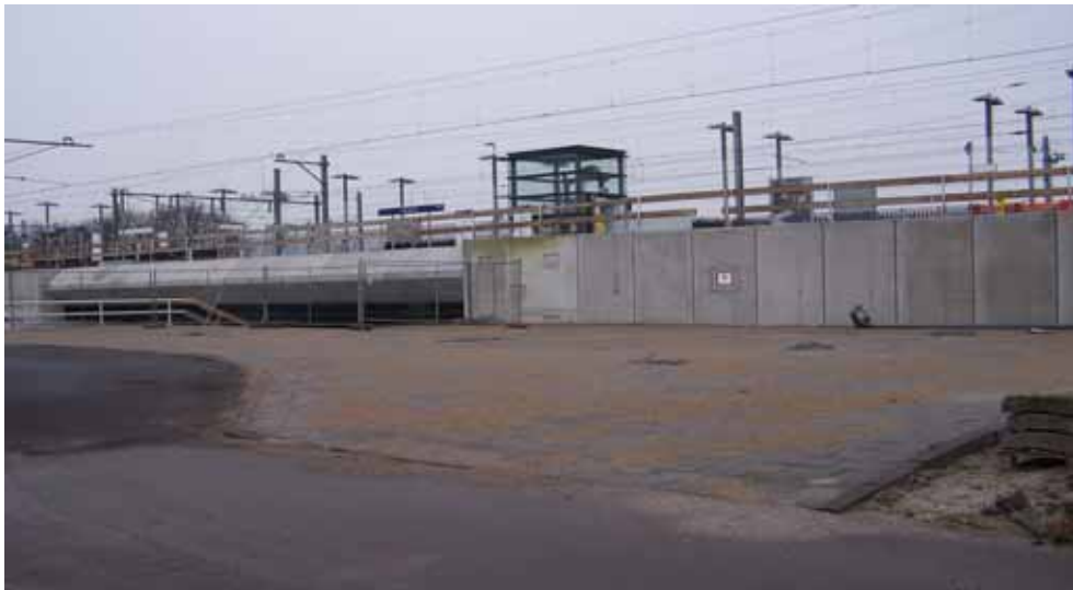
Foto 5.4 Station Forepark december 2006
