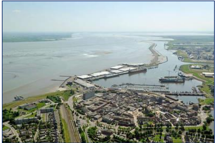
Fig. 6: The harbour of Delfzijl (Source: Provincie Groningen, 2012)
