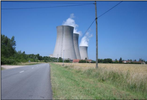
Fig. 7.1 Dampierre (Loiret) Nuclear Power Plant
