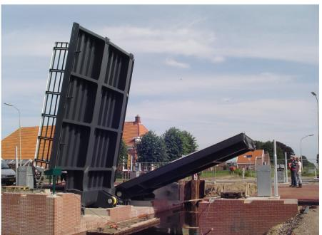
Figure 7: 2006: Central dam in Kiel-Windeweer is replaced by a modern drawbridge. In the background the old dam is still visible (source: kiel-windeweer.nl)
