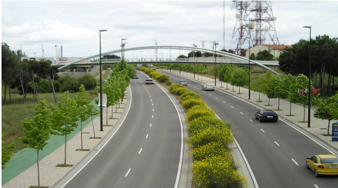
Figure 5.10: Restored road infrastructure (Auke Vlonk)
