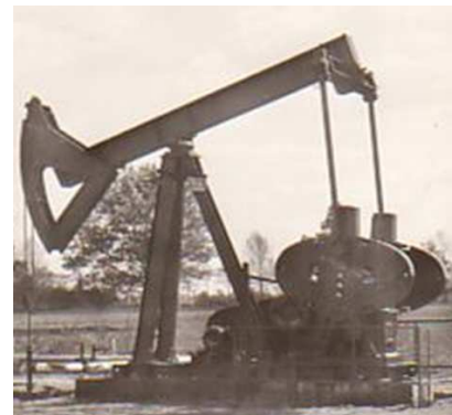
Figure 5 Pumpjack of the NAM in Schoonebeek source: Ten Cate 2007
