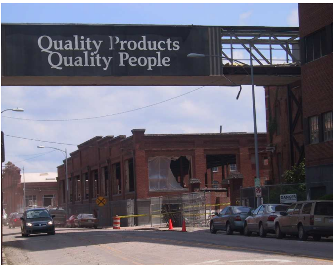
Figure 12 Liggett & Myers under construction (2007) Foto by G. van der Pol
