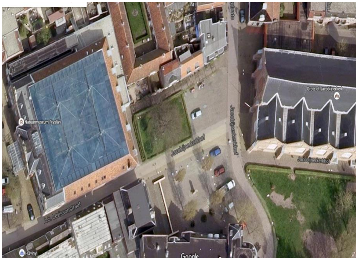
Figure 3: Areal overview of Holocaust Monument and immediate vicinity (source: google maps, 2016)
