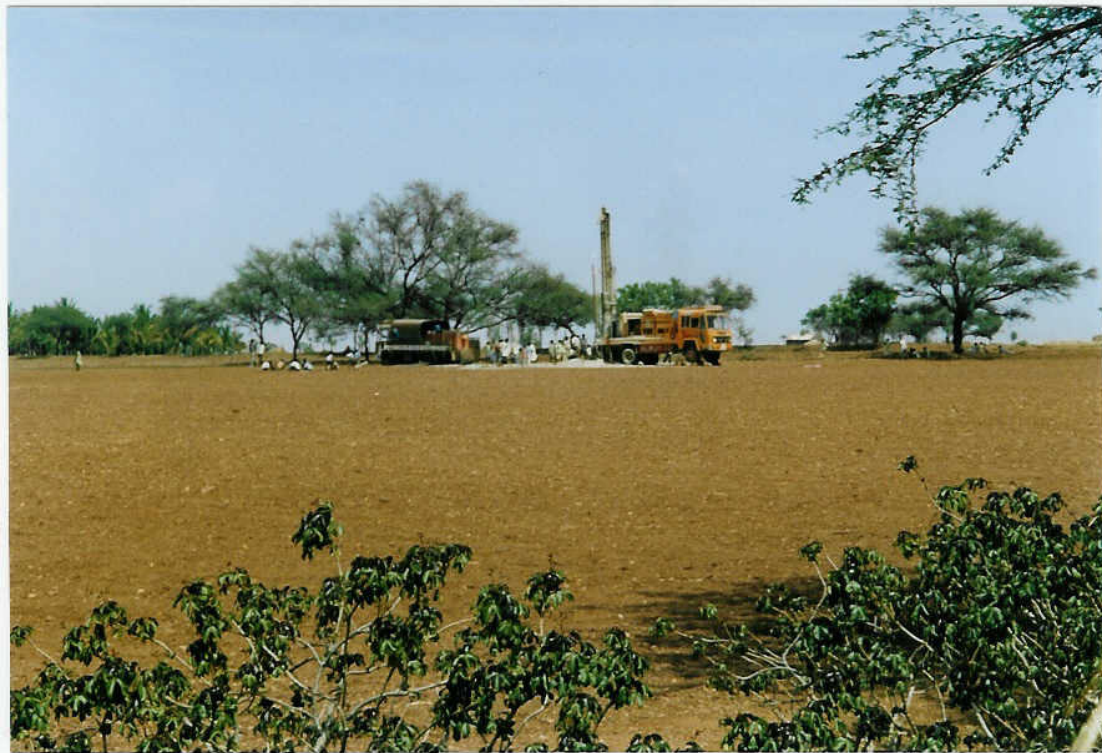
Digging of a bore-well
