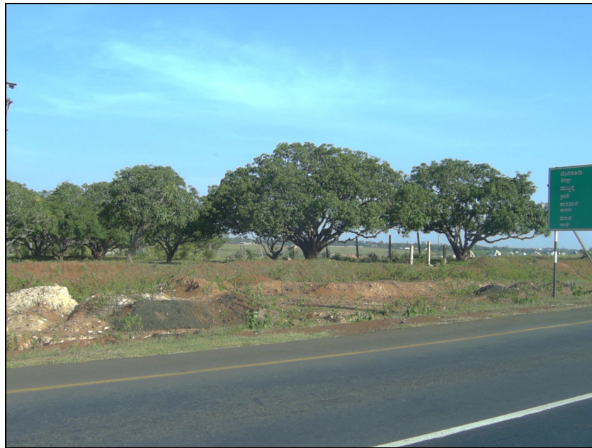
Figure 5.8 The by-pass cutting through old mango-orchards, west of the twin-city (source: fieldwork)
