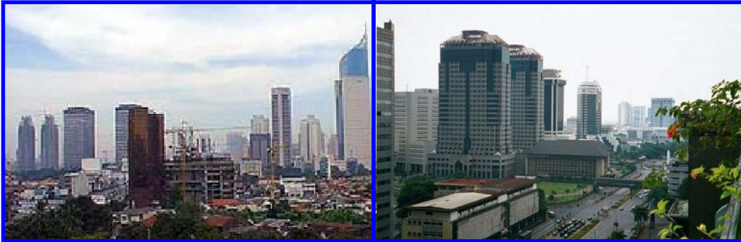
Figure 16 High Rise Building in the Central Area of Jakarta
