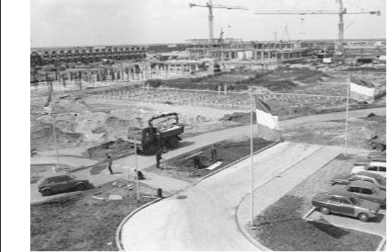
Figure 5 – Construction of Almere Stad in 1980 (source: Flevoland’s archive).
