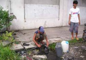
Figure 3.5: a) Spaghetti connection of BACIWA lines; b) Illegal water tapping in the city of Bacolod.
