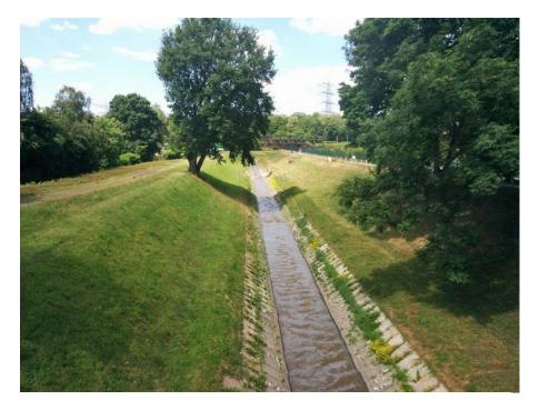
Figure 4: One of the Emscher tributaries that was transformed into an open sewage channel (Source: Paulina Budryte)
