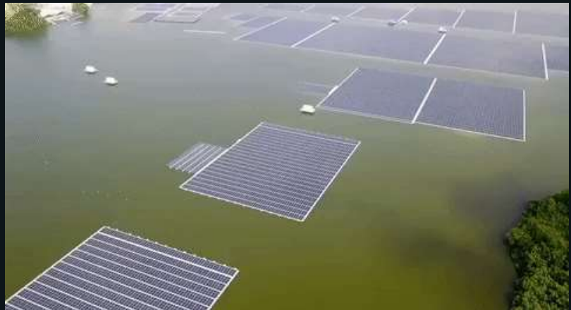
FIGURE 17 FLOATING SOLAR FARM SINGAPORE (TAN, 2021).
