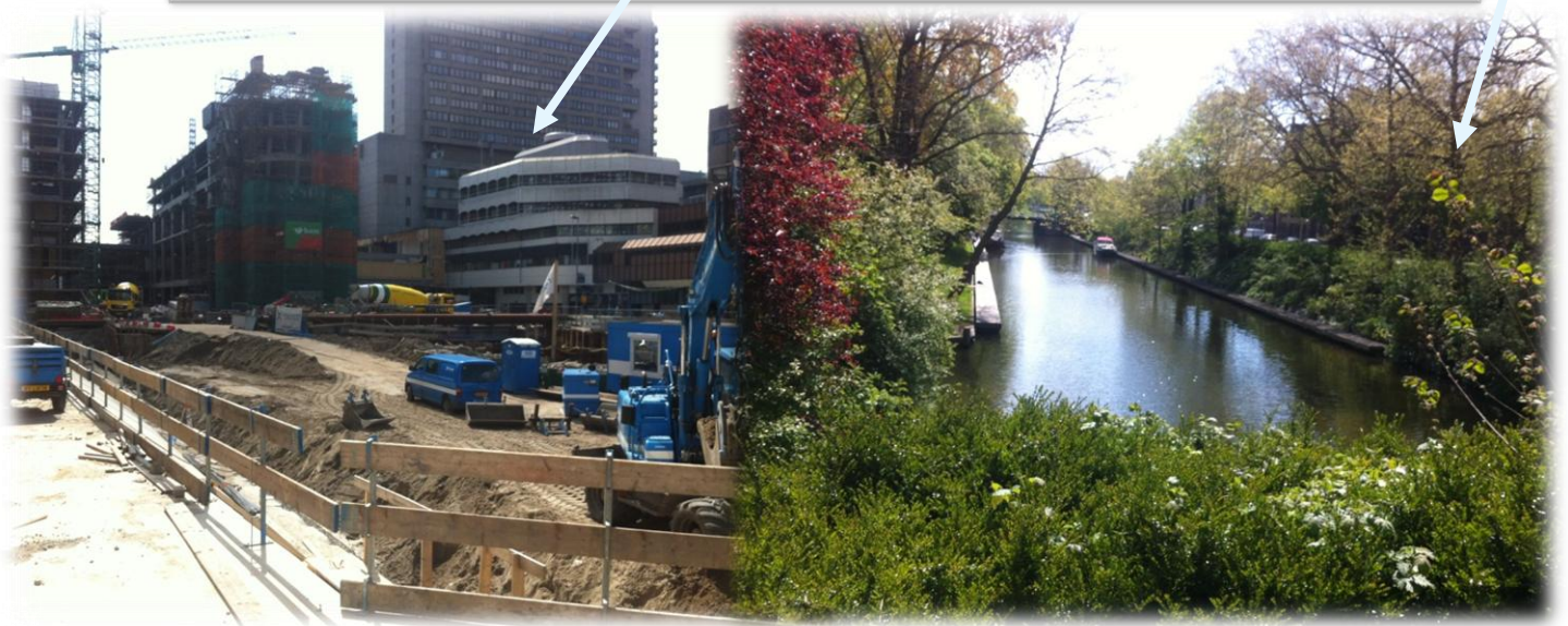
Catharijnesingel under construction
