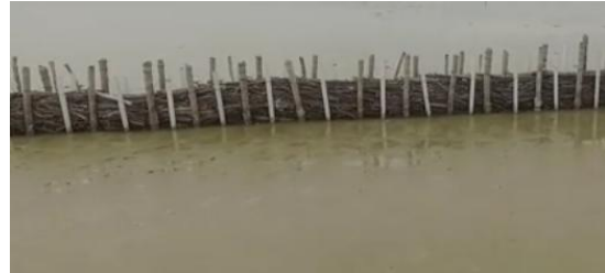
Figure 8: Semi-permeable dam made out of bamboo branches (WitteveenBos, 2016)
