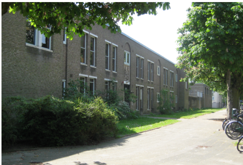
Figure 4: Front site of several apartments of the Amunshofje behind there is a courtyard (Nul20, 2022)
