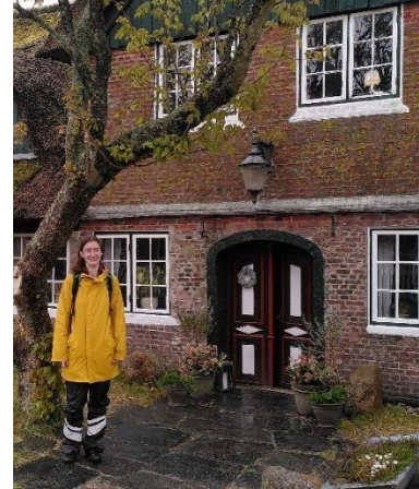
Figure 1 An example of a monumental house: the Sønnerho Kro. Picture from the author.
