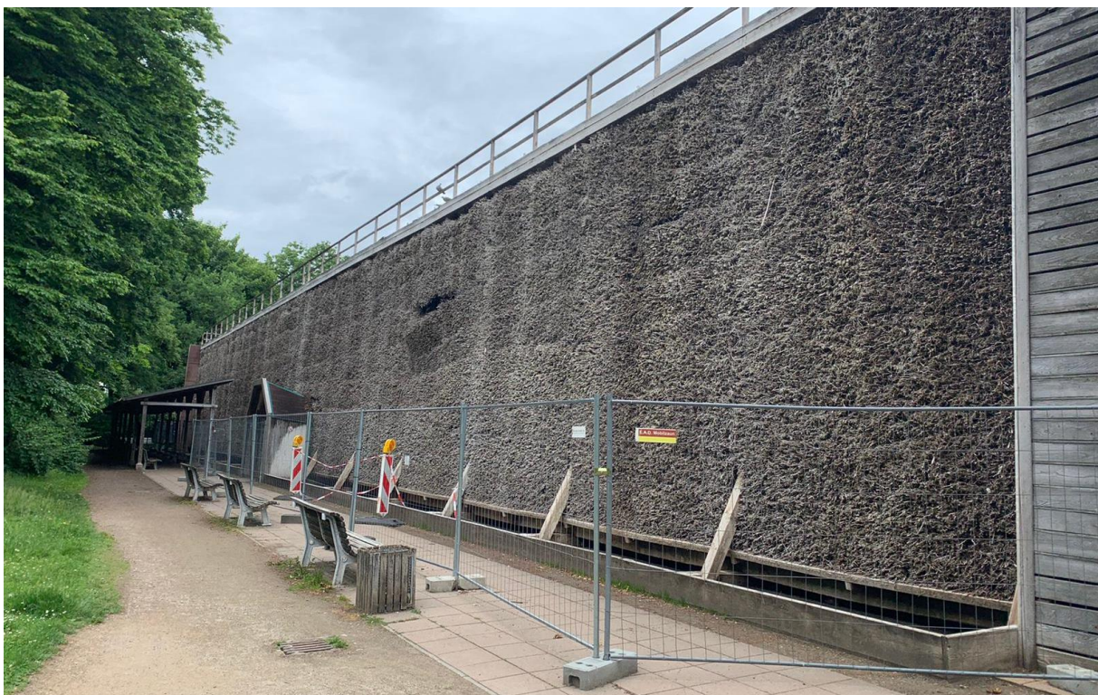
Fig. 8: Salina out of order, waiting for repair, 2022.
