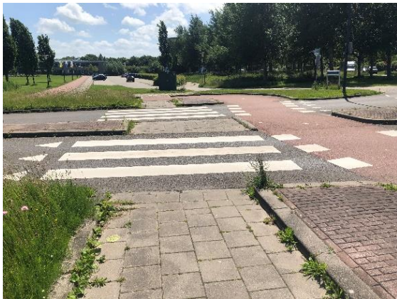
Figure 7: The roundabout at the Foudering and the Wittemar (picture taken by Author)
