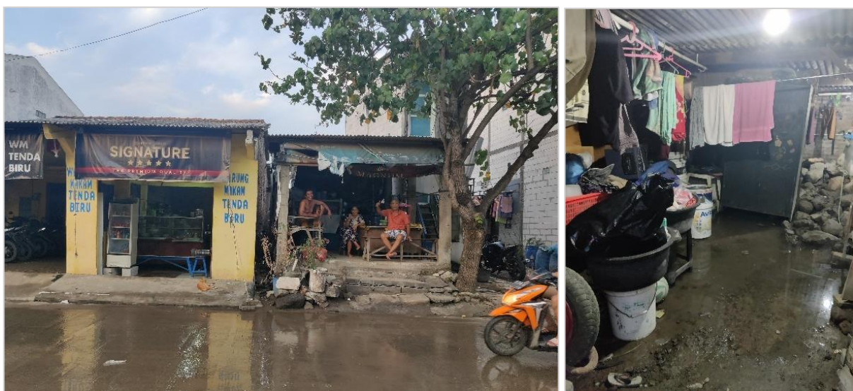
Figure 4.5: Frontside (left) and inside (right) of an house between high and ebb-tide (photos by author)
