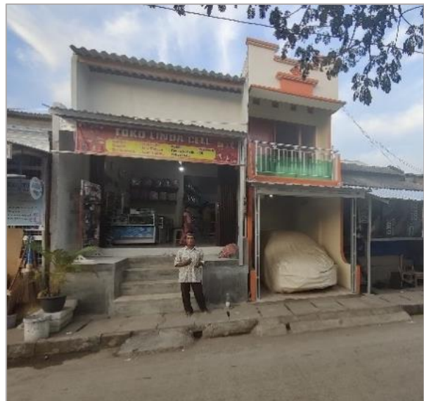
Figure 4.10: Raised house levels (photo by author)
