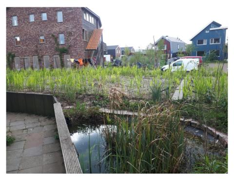
**Figure 7**: Halophyte water-filter system in IEWAN. Gray water from IEWAN is filtered via this system and re-used to flush toilets.
