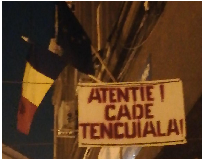
Figure 11: Sign pointing out the danger of falling debris from buildings
