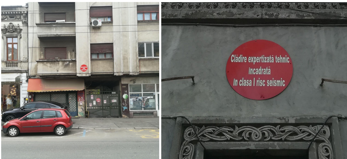
Figure 9: Buildings categorized under risk class 1 with the distinctive red dot symbol (Source: Author)
