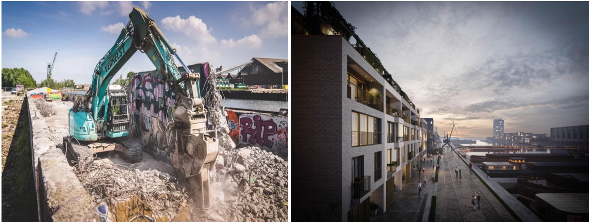
Figure 18 & 19: Demolition and renewal in Oude Dokken / Source: Selfslagh, 2014; Immoweb, z.d.
