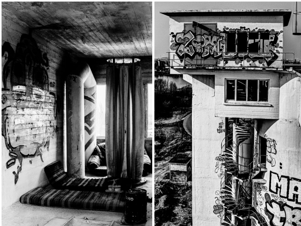
Figure 6 & 7: The Concrete Factory in Ghent / Verstraete (z.d.)
