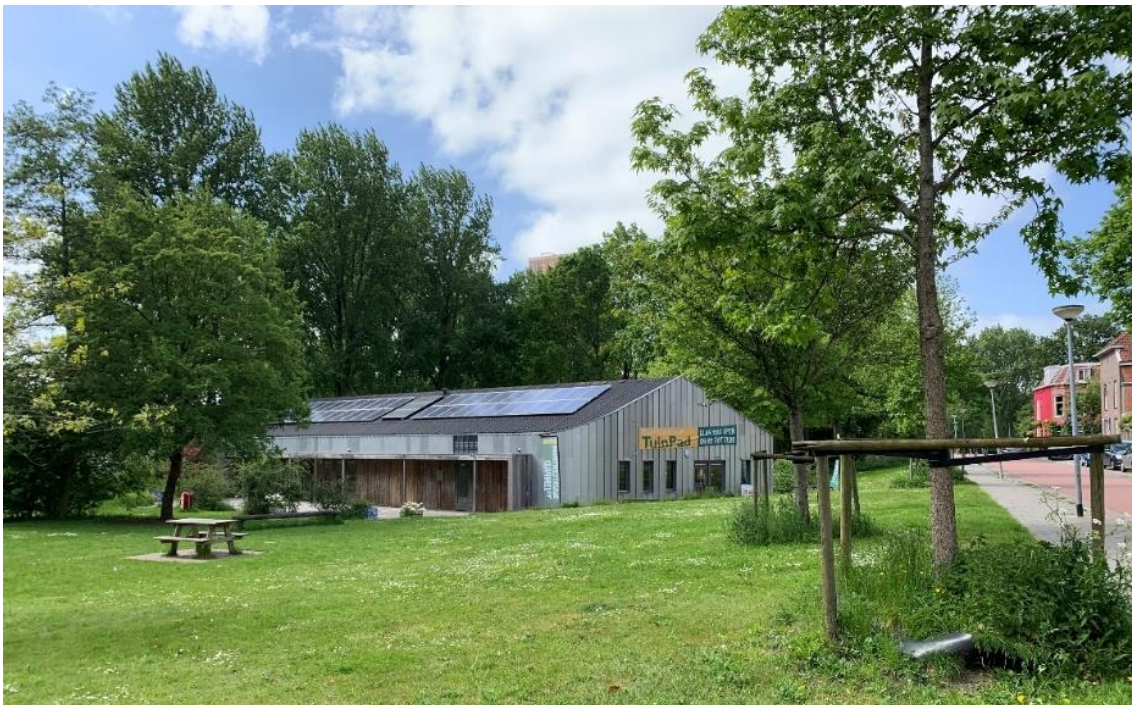
Fig. 7 New community center at Bessemoerpark (Author, 2023)
