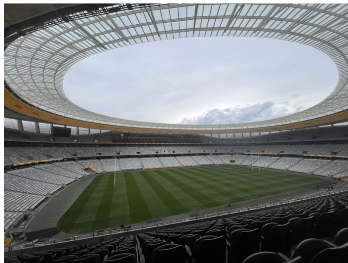
Figure 7: DHL stadium (former Cape Town stadium) from the inside (Author photo)
