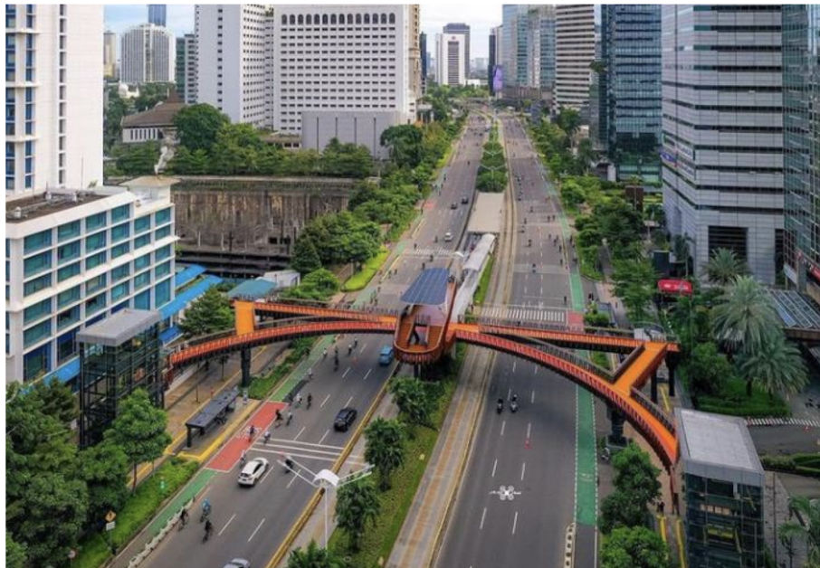
Figure V. Pedestrian Bridges (The Provincial Government of DKI Jakarta, 2022, p.379)
