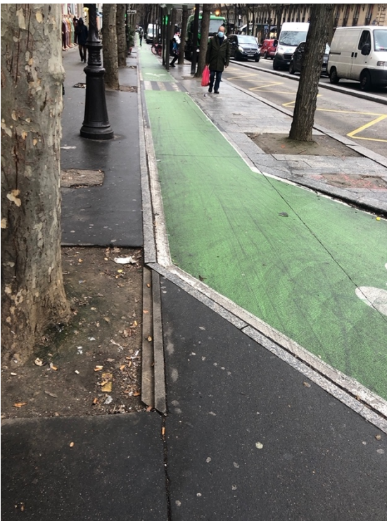
Figure 24: Dedicated protected cycling lane, the "holy grail" of cycling infrastructure in green, Paris, photo by author (2023)
