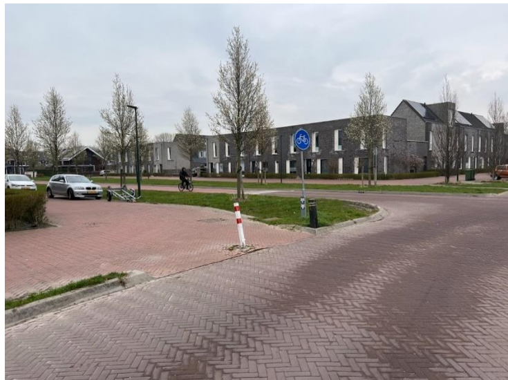
Picture 4: Physical separation between cars and bicycles on main access road in Harinxmaland
