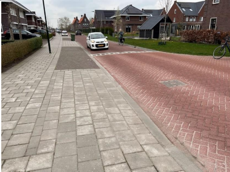
Picture 5: Wide sidewalk on main access road in Harinxmaland
