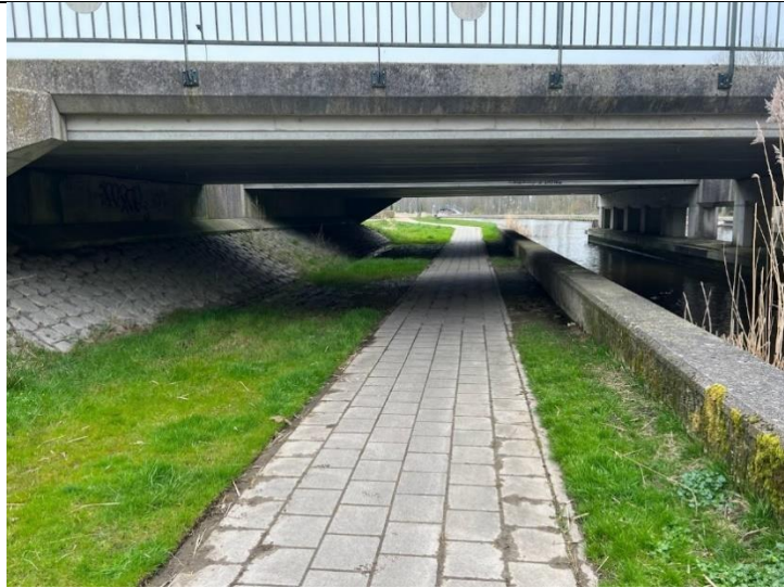
Picture 21: Grade-separated crossing of N354 road near Harinxmaland (only sidewalk, not connected to main bicycle routes)
