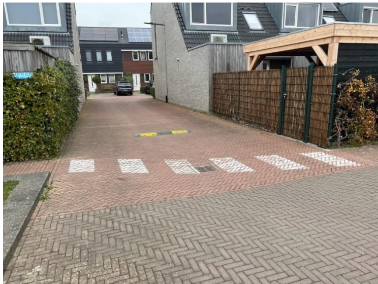
Picture 12: Provisional speed bump and zebra crossing in Harinxmaland
