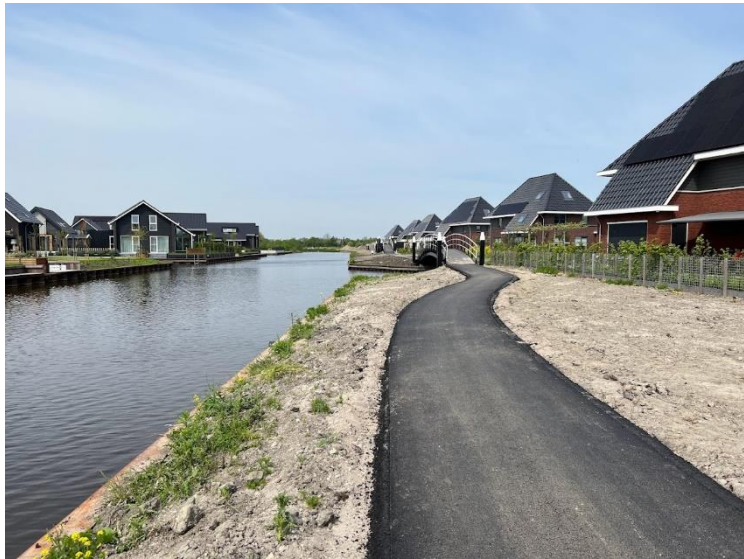
Picture 15: Not yet finished main cycling path through Harinxmland
