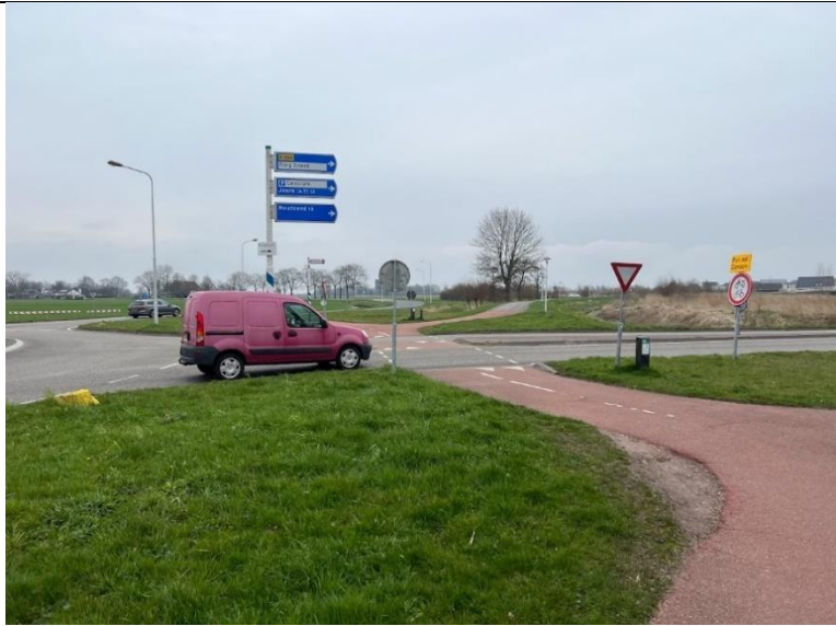
Picture 23: Unregulated level crossing of provincial 80 km/h N354 road (Stadsrondweg-Oost) near Houkepoort
