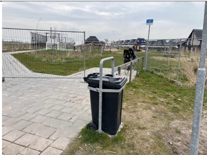
Picture 38: The large playground in Harinxmaland has a bicycle stand and is accessible by sidewalks and the new cycling path. No cars nearby.
