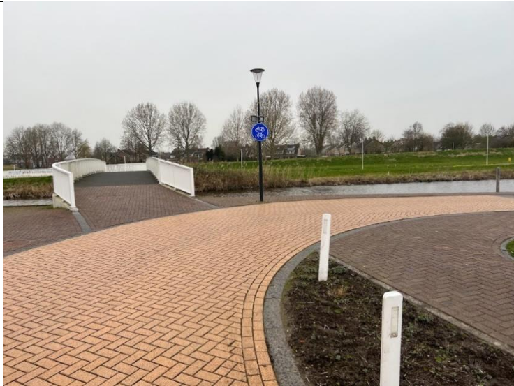
Picture 19: The slow traffic routes in Houkepoort are in general well-maintained
