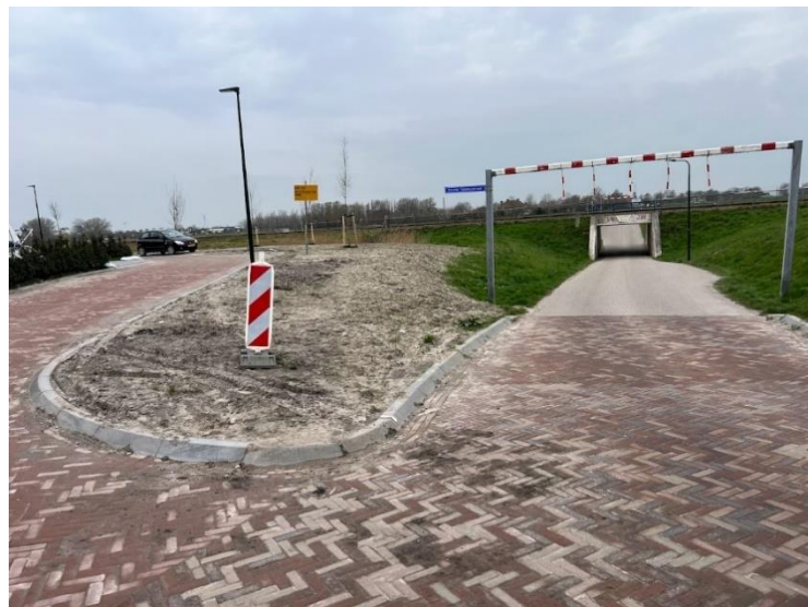
Picture 22: Grade-separated crossing rail line Leeuwarden-Stavoren and connection between Harinxmaland phase 1 and 2
