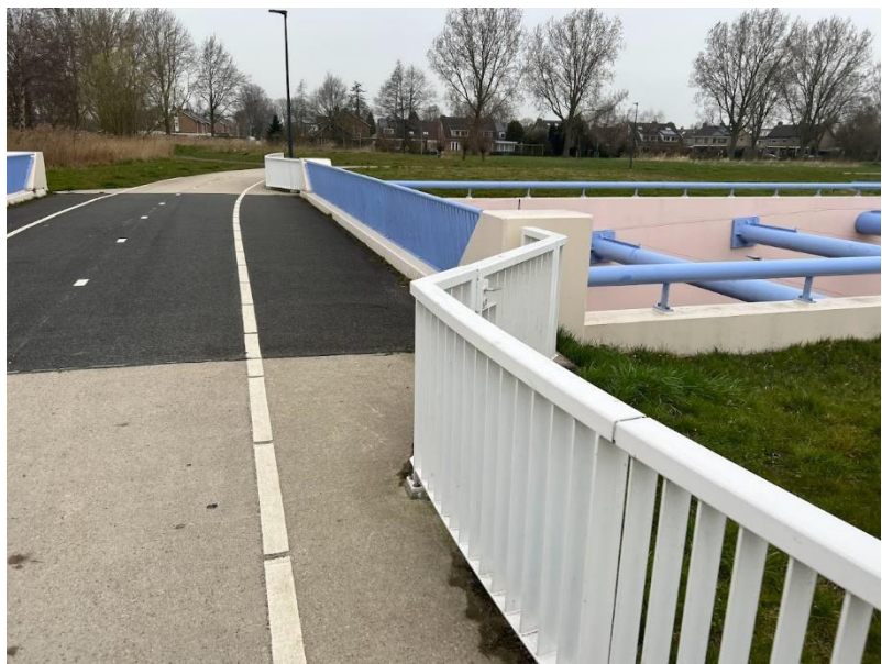
Picture 24: Grade-separated crossing of N354 road (bicycle path, connected to main bicycle route)
