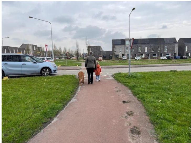
Picture 20: Unregulated level crossing of provincial 80 km/h N354 road (Stadsrondweg-Noord) near Harinxmaland
