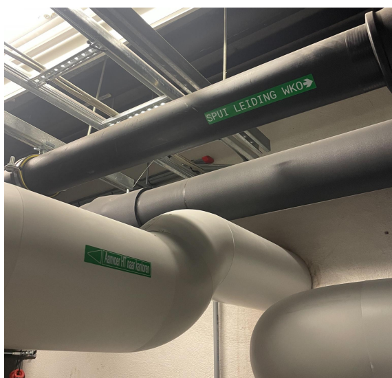
Figure 22: Pipe network with insulation
