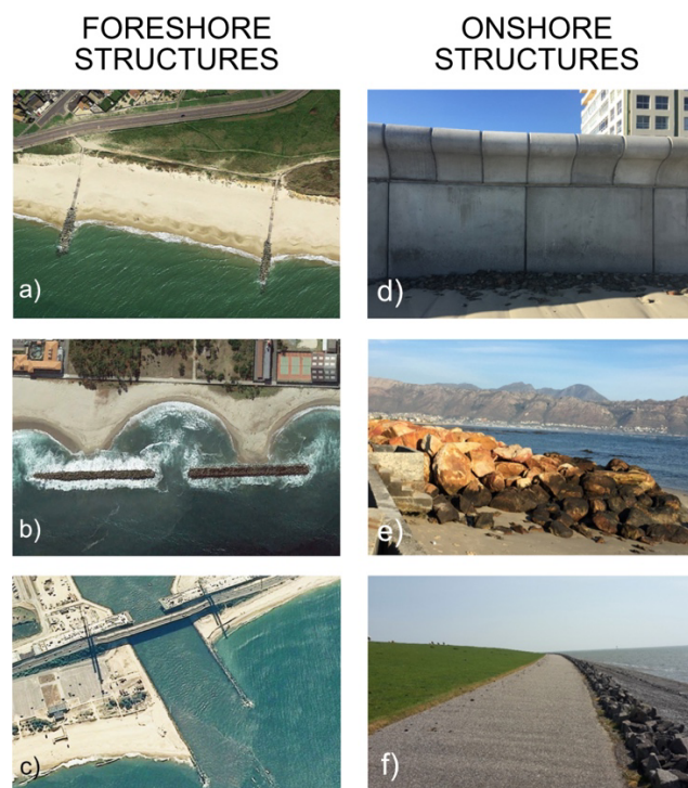
Figure 4: Traditional coastal protection structures (adapted from Schoonees et al., 2019)
