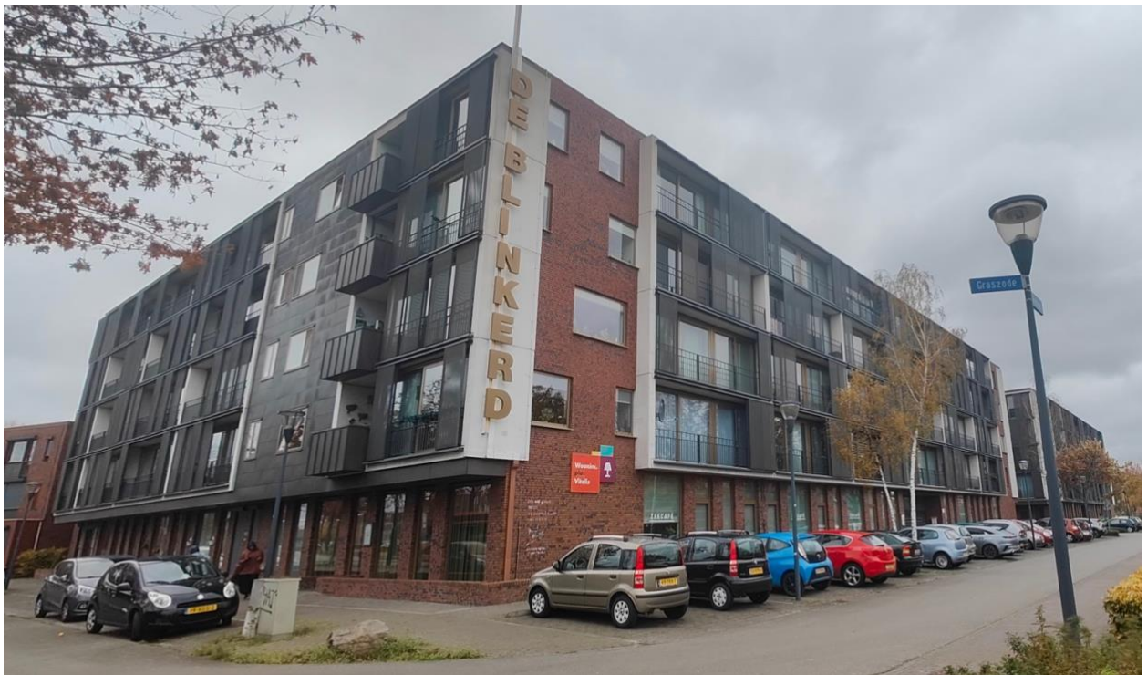
Figure 10: Apartment building in the center of Meerhoven-Grasrijk.
