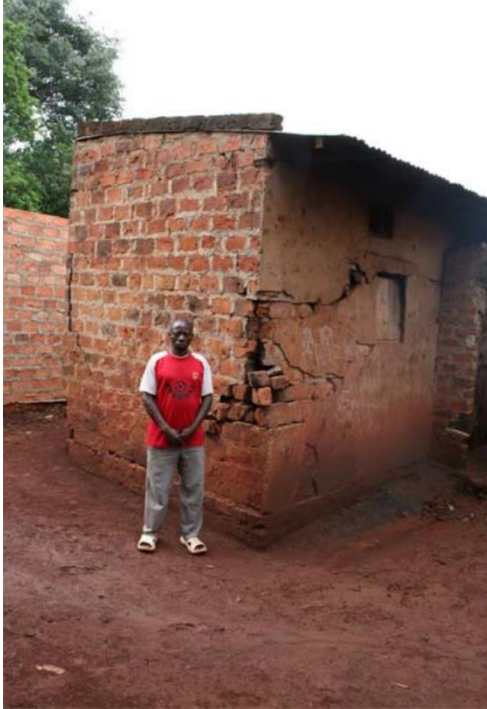
Figure 10: Impacts on local housing by BEL-coordinated rock blasting (IRM, 2009, p.14)
