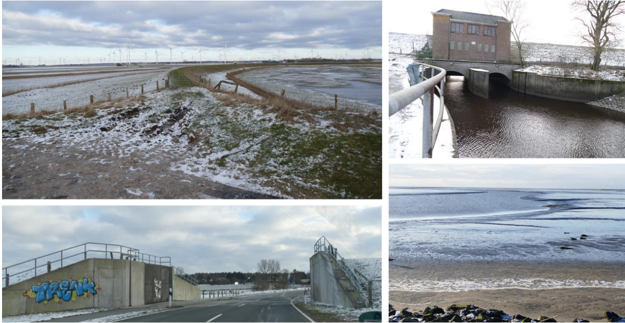
Figure 14: Impressions of the mainland of SH Wadden: old dike lines with roads passing through them, sluice (top left) and dredged channel (bottom right) for inland drainage. Source: Author.
