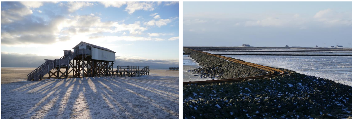
Figure 20: Accommodating measures. A house built on stilts (left) in St. Peter-Ording and a dam leading to the Hallig Nordstrandischmoor with its typical terps (right). Source: Author.
