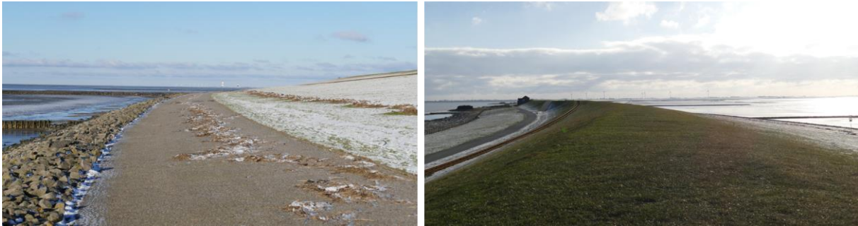
Figure 16: Climate Dike with a flat and wide dike crest to improve dike reinforcement in the future. Source: Author.
