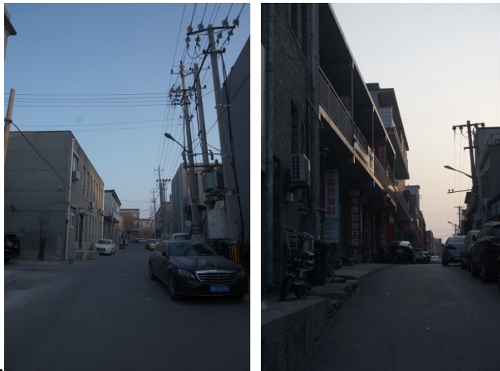
Figure 7-3 Landscape before renovation
