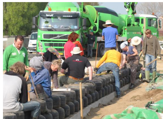
Figure 1 - Self-build with walls constructed from tires (Vereniging Aardehuizen, 2022).
