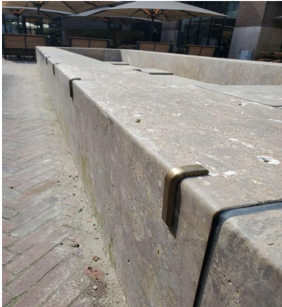
Figure 49: A new skate-stopped bench in the Waagplein next to the Grote Markt (Author, 2024)
