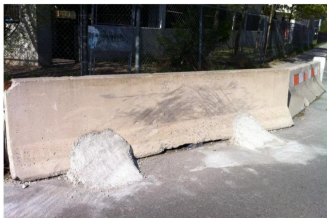
A simple DIY addition to a jersey barrier (Gopal, 2012)
