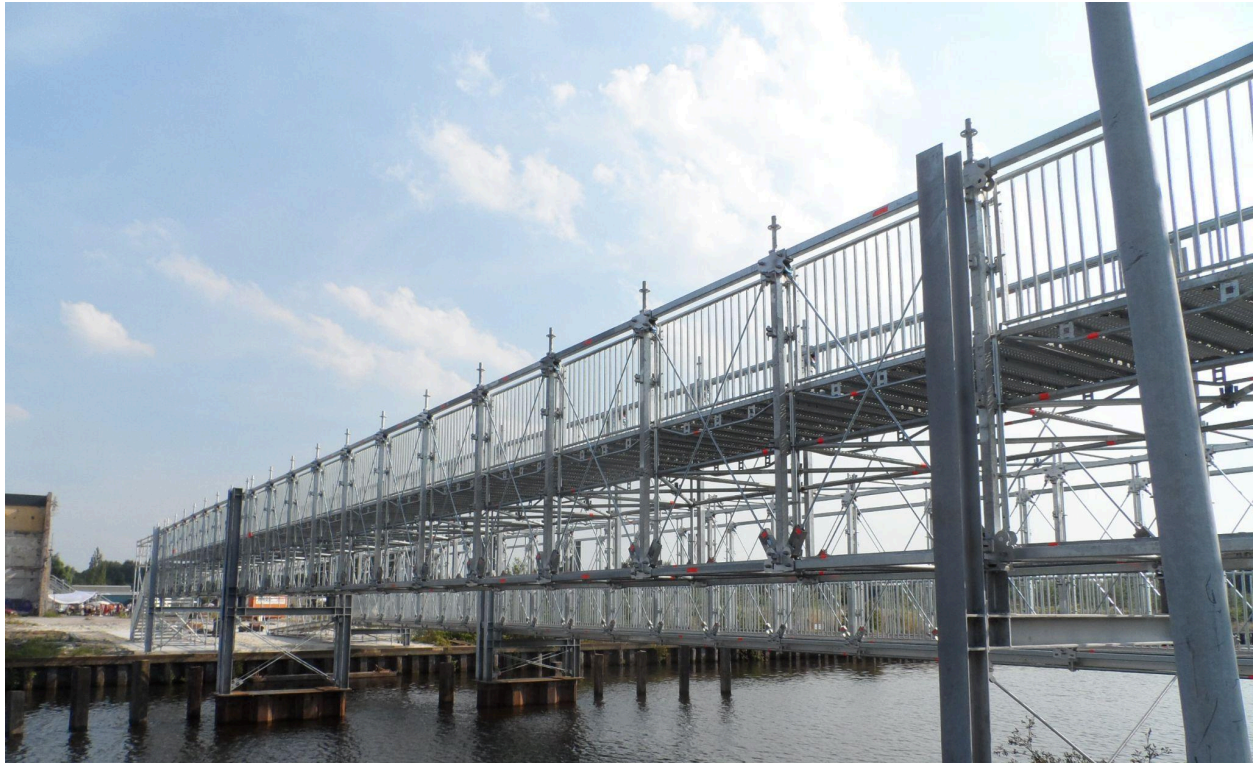
Figure 6: New temporary bridge across the Hoendiep (Afdeling Kunst & Cultuur, 2014)
