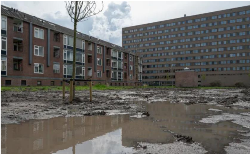
Figure 2: Problems with excess water. (FocusGroningen)
