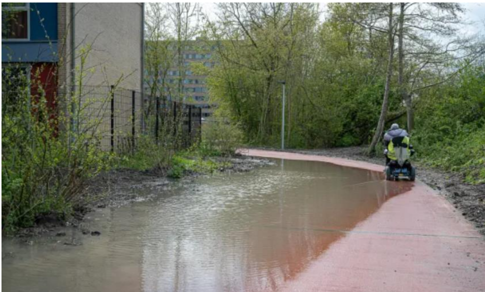
Figure 7: excess water resulting in flooded pavements. (FocusGroningen)
