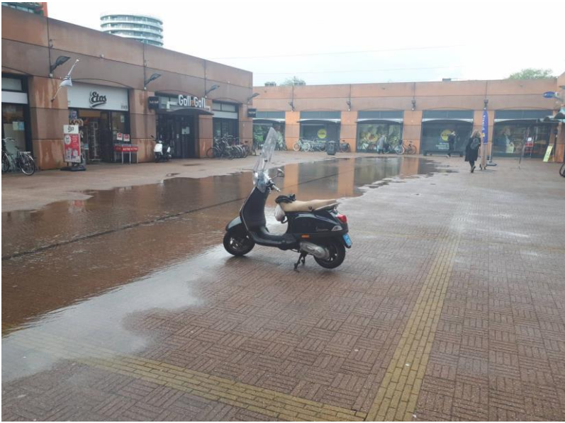
Figure 1: Problems with surface water run-off. (Hanze University).
