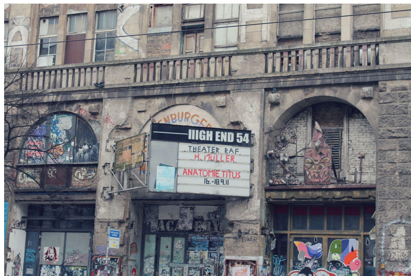
Figure 21 (top): Entrance Fotografiska (Bolon, 2024) & Figure 22: Entrance Tacheles (Canale, 2015)
