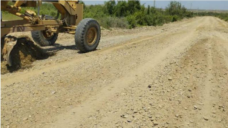
Figure 6: Road between Talara and Lobitos (Source: Estado Peruano, 2023)
