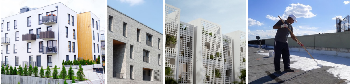
Figure 11 impressions of high albedo materials on building surfaces (Roidou, 2021; van der Laan, 2024)
