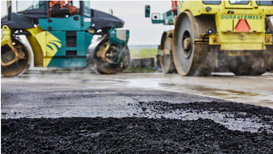
Figure 9: Test of asphalt Roof2Roof at construction site (Dura Vermeer, 2024a)
