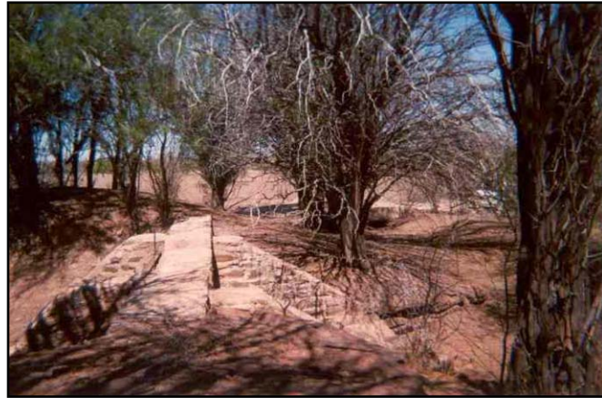
Picture 5.10: Water intake of irrigation fields in the background (picture by author).
