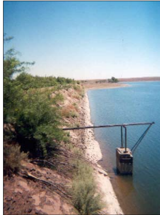
Picture 5.5: The valve that feeds the irrigation system (picture: author).
